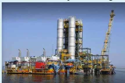
Picture 2.1: Kivu watt power station
